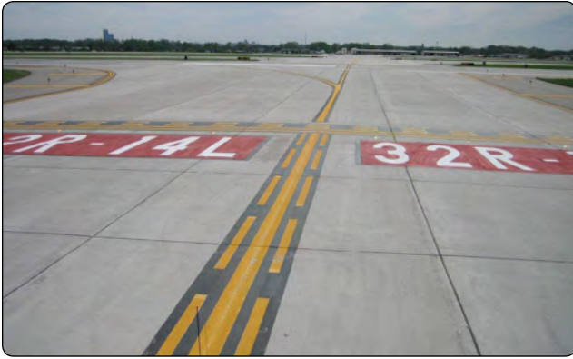
Figure 14-12. Surface painted runway holding position signs for Runway 32R-14L along with the enhanced taxiway centerline marking.
