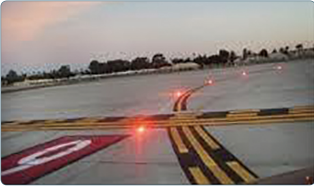
Figure 14-35. Runway Entrance Lights (REL).
