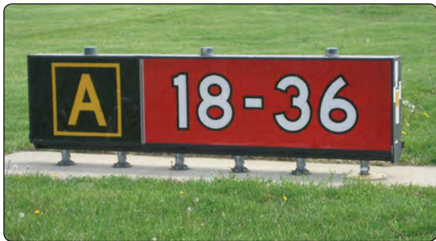
Figure 14-10. Runway holding position sign at a location other than the takeoff end of Runway 18-36 with collocated Taxiway Alpha location sign.
